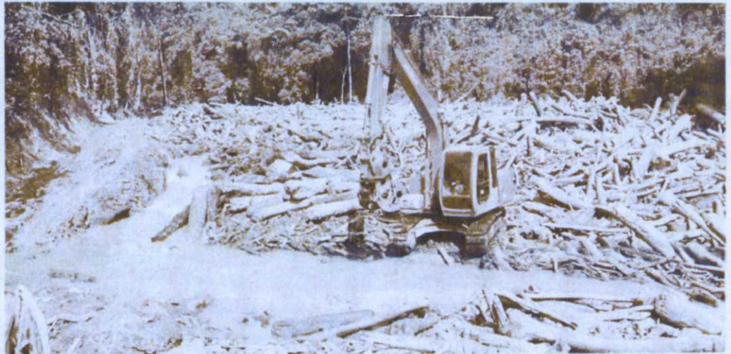
Work in progress: An excavator being used to clear the timber debris in Sungai Liwagu where the Ranau water treatment intake point is located.
